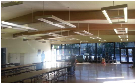
Cafeteria in need of upgrade and expansion.
