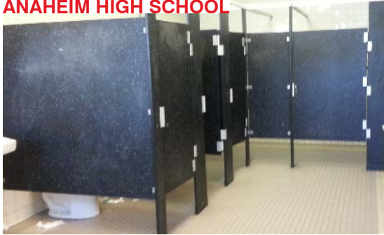
Restrooms need to be upgraded.
